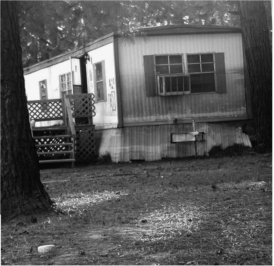
Figure 2. Flooded mobile home in a densely vegetated trailer park on the floodplain, just north of the Tar River, Greenville, North Carolina. The high-water mark reaching the middle of windows is clearly shown on the side of the mobile home.
